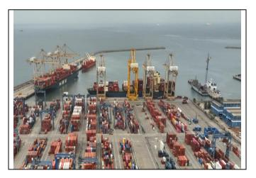
There are two container berths and one multi cargo berth located in the northern part of the harbour , lengths of berths are B  $1-350\mathrm{m}$ , B  $2-360\mathrm{m}$ , B  $3-294\mathrm{m}$  and depth alongside is 16.0m. There is an old seawater intake/discharge facility for the Chennai Petroleum Corporation Limited (CPCL), to the south which is linked to shore by a  $500\mathrm{\ m}$  mtrs long causeway.
